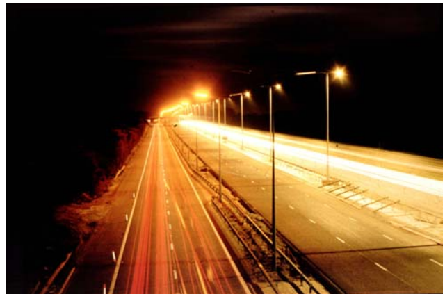
M5 widening LPS and HPS Full Cut Off Ken Sheldon and Chris Baddiley, CfDS Image Archive
