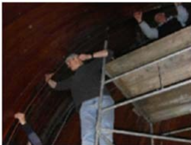
Fig. 2. Fitting the runners for the sunshade. (ML)
